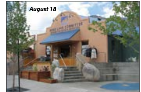
Above: Once the concrete Mono Lake map was completed, the storefront got Trex decking, the wheelchair lift, drinking fountain, redwood pergola, and planters.
