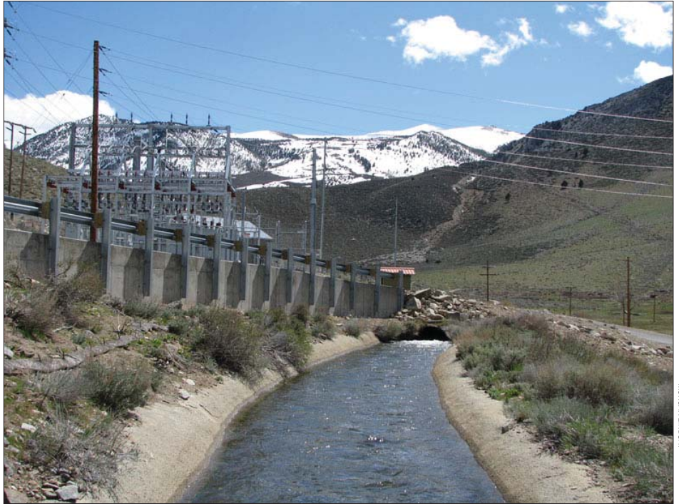
Mill Creek's water leaving the Lundy hydropower plant.
