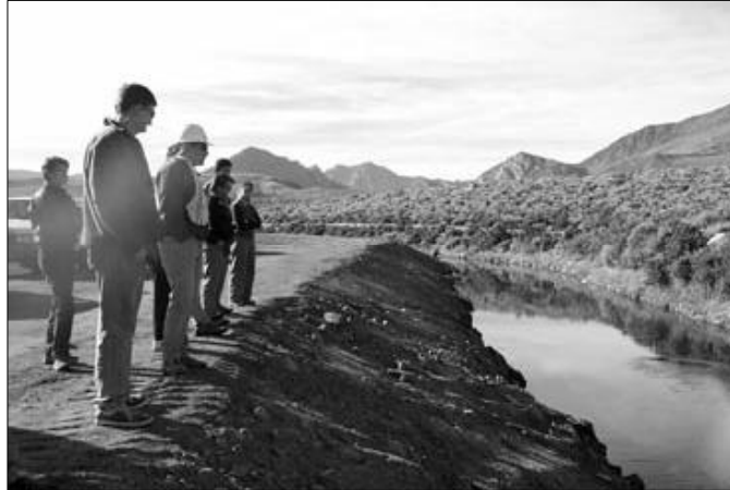
Committee and DWP staff out at the Rush Creek return ditch. Peak flows are expected to raise the water level five feet above the level in this photograph—necessitating the rehabilitation project.
