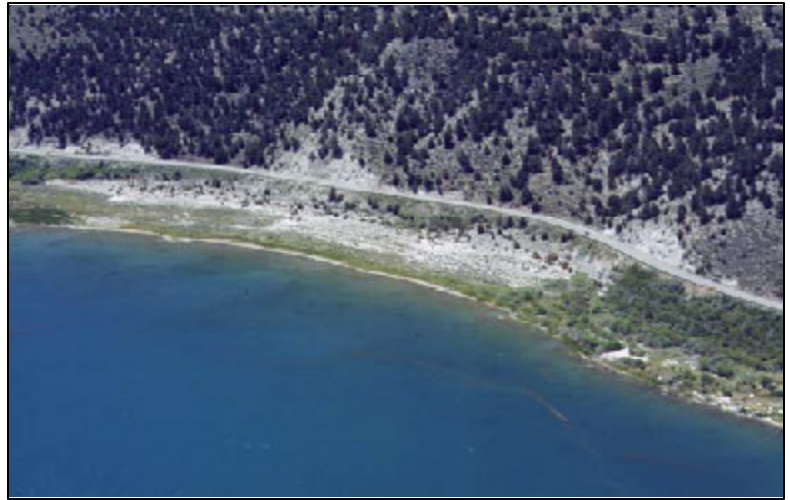
Hwy 395 along Mono Lake in Caltrans' Mono Lake Widening Project area.
