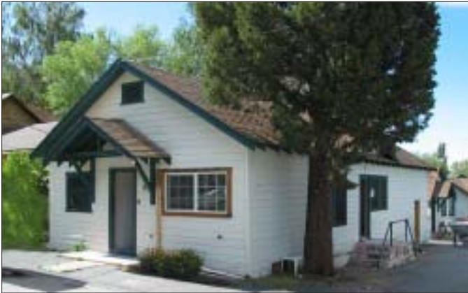
The Mono Basin Field Station Building in Lee Vining.
