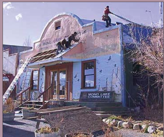
The new roof on the Mono Lake Committee headquarters.
