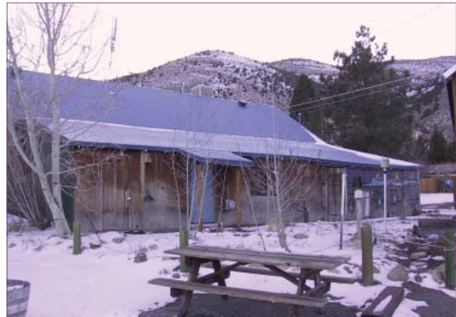
December 11, 2006: The new roof is strong corrugated metal in a beautiful shade of blue, and best of all, no more leaks!
