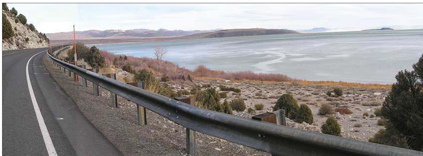
Caltrans' guardrail project for motorist safety has been completed without any lake-disturbing activity. The Committee continues to advocate for a more visually appropriate guardrail for this section of Hwy 395 that runs through the Mono Basin National Forest Scenic Area.
