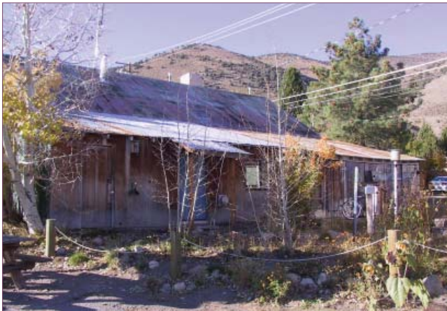
November 11, 2006: After over 40 years of sheltering the building, the Committee's old roof was full of holes and patches.
