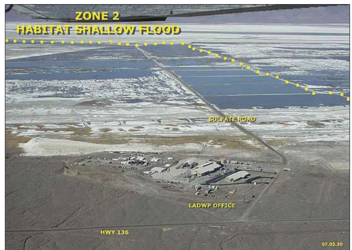
Sulfate Road at Owens Lake with a large expanse of habitat-creating shallow flood dust control.
