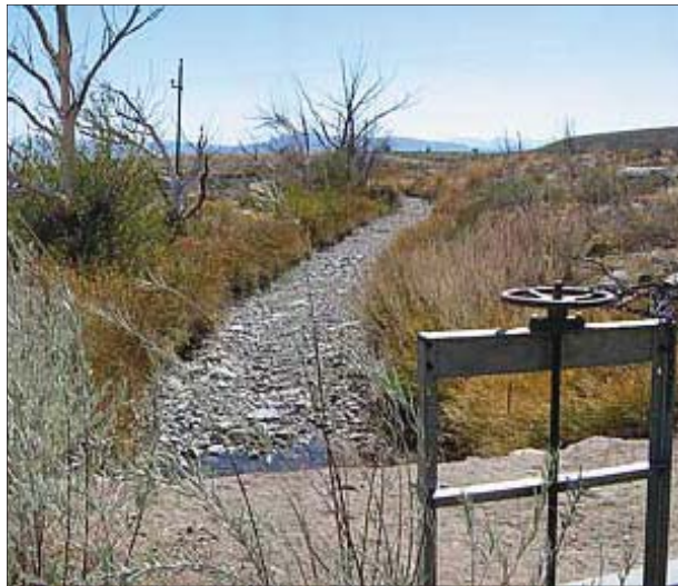
The Mill Creek return ditch.
