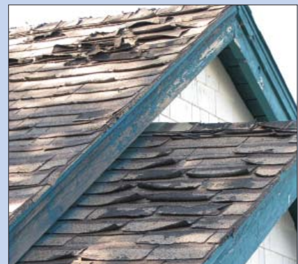
The Field Station roof is ready for repair!
