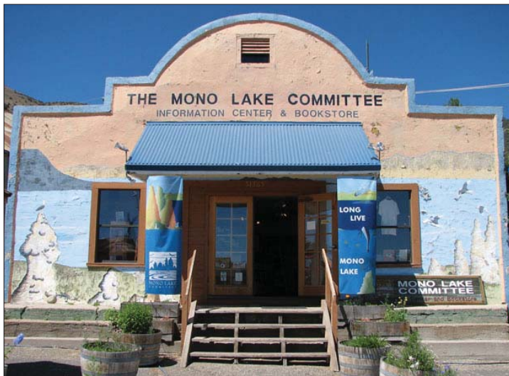
The Mono Lake Committee Information Center & Bookstore façade will be repaired and refreshed this year.
