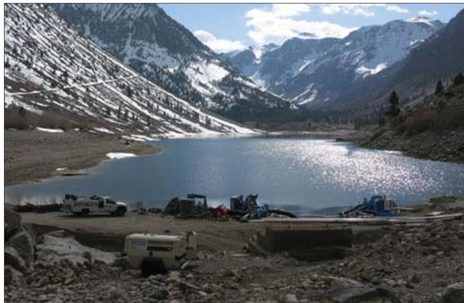
The Lundy Dam repair project.
