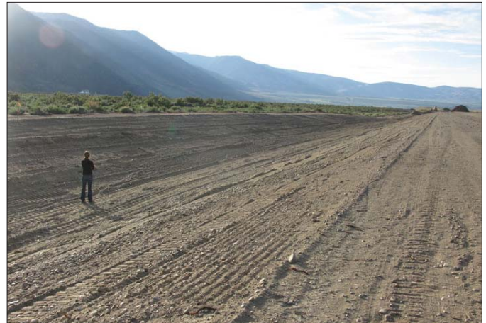
The excessively large drainage ditch west of the runway contributed to the size of the stockpile that obstructed views from Lee Vining.
