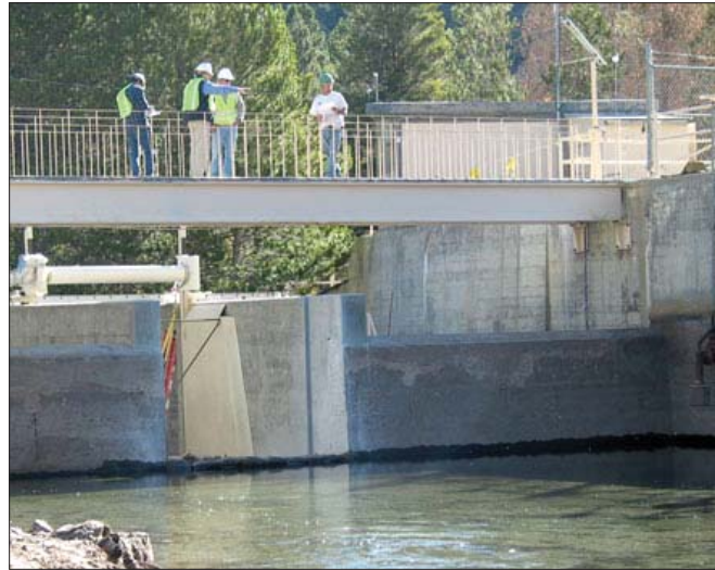
Structural upgrades on the Lee Vining Creek diversion facility allow DWP to better meet State Water Board restoration requirements.
