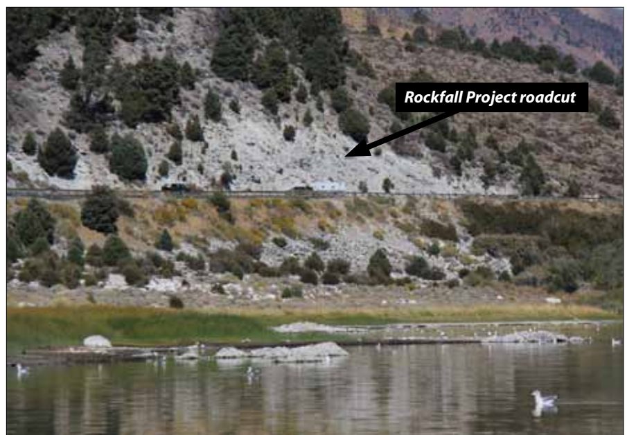
The Rockfall Project slopes are located close to Mono Lake. One of the Committee's concerns is that slope erosion can produce sediment that impacts adjacent wetlands and the lake.
