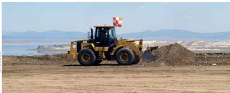
In August, earthmovers removed 2,000 cubic yards of soil from the stockpile at the Lee Vining Airport—reducing its height by one foot and improving the view of Mono Lake from town.
