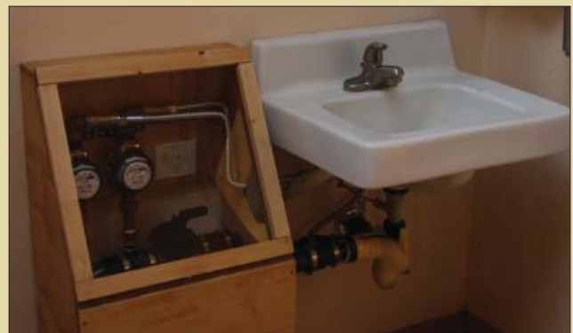
The Eastern Sierra's first commercial greywater recycling system was installed in the Mono Lake Committee Information Center & Bookstore bathroom!
