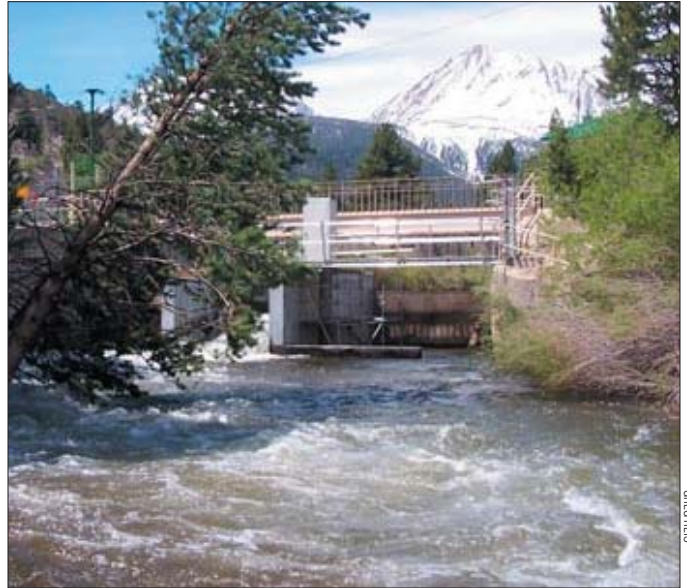
The upgraded Lee Vining Creek sediment bypass facility no longer blocks sediment needed for fish habitat and new vegetation, but allows it to pass downstream.
