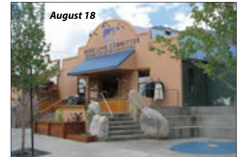
Above: Once the concrete Mono Lake map was completed, the storefront got Trex decking, the wheelchair lift, drinking fountain, redwood pergola, and planters.
