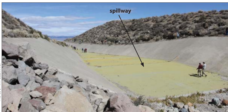
With the new Grant Outlet constructed, this view will show new flow gates installed in a notch in the existing concrete. When high flows are required, the notch will carry water to Rush Creek.
