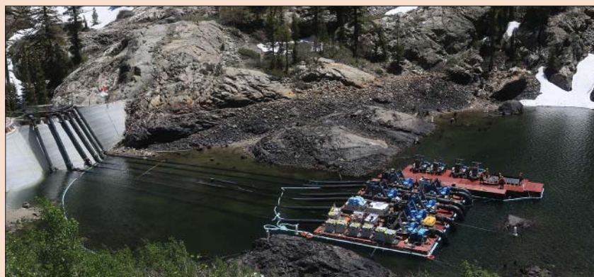
SCE is required to keep its Rush Creek watershed reservoirs at 50% capacity—this year, that involved moving water over Agnew Dam using pumps on barges.
