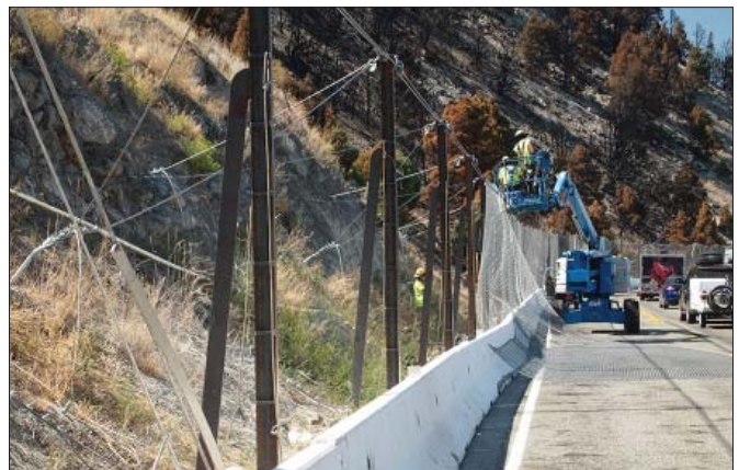
Phase one of the Lee Vining Rockfall Safety Project along Highway 395 west of Mono Lake was completed on time last fall. Safety measures installed after the Marina Fire, including white concrete barricade and heavy duty high fencing, will remain until the slopes are secure.
