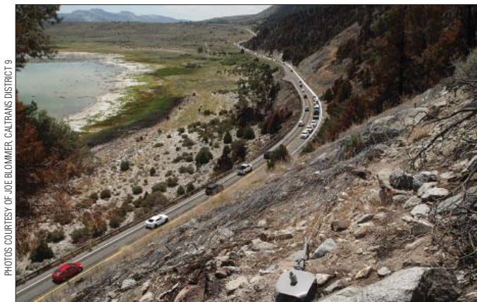
Phase one of the Lee Vining Rockfall Safety Project along Highway 395 west of Mono Lake was completed on time last fall. Safety measures installed after the Marina Fire, including white concrete barricade and heavy duty high fencing, will remain until the slopes are secure.
