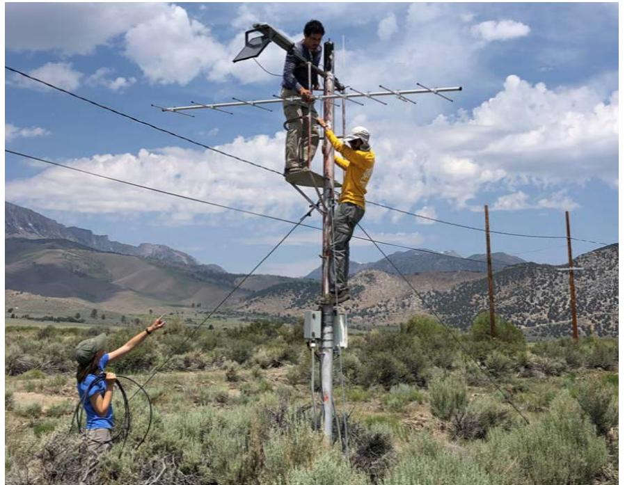
*Building a Motus data receiving station for wildlife tracking using radio telemetry.*
