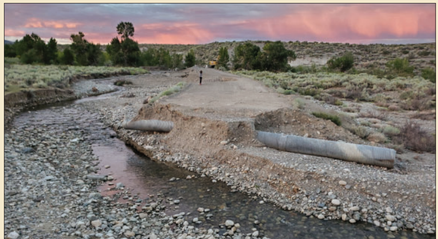
Mill Creek's peak flows had to be diverted around too-small culverts at Cemetery Road.
