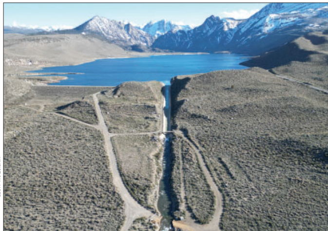
Use of the Grant Lake Reservoir spillway can mitigate DWP's inability to deliver required Rush Creek restoration flows because of a broken 89-year-old aqueduct intake valve located 80 feet underground.
