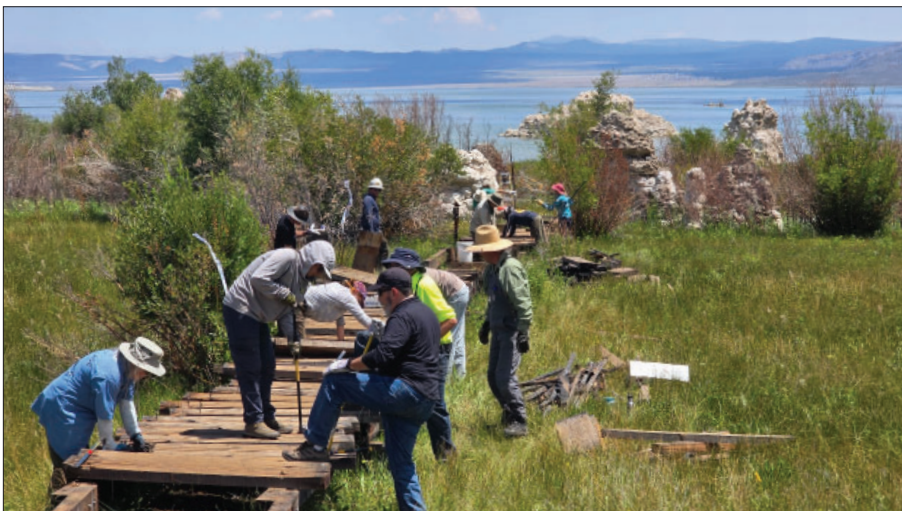
After the Inn Fire was contained, 75 people worked to remove the entire damaged State Reserve boardwalk at County Park, readying the site for a new, non-combustible boardwalk.
