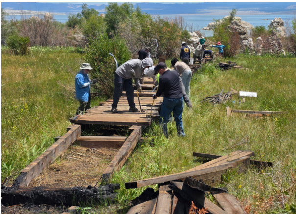
Removing the burned boardwalk has expedited State Parks' ability to replace the boardwalk at this beloved visitor site.
