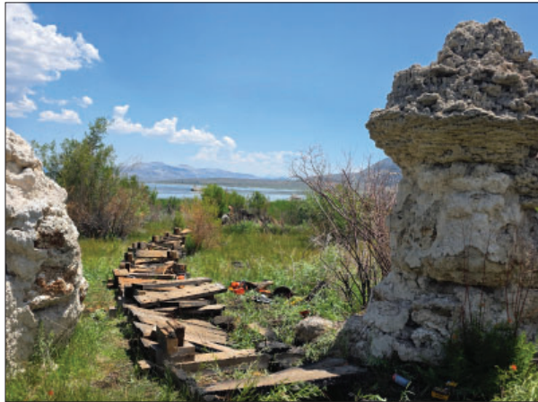
Replacement of the State Reserve boardwalk at Mono Lake County Park will not happen until after summer this year.
