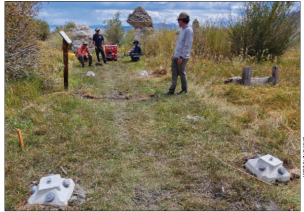
Construction of the State Reserve boardwalk below Mono Lake County Park is underway, with plans to reopen in 2027.
