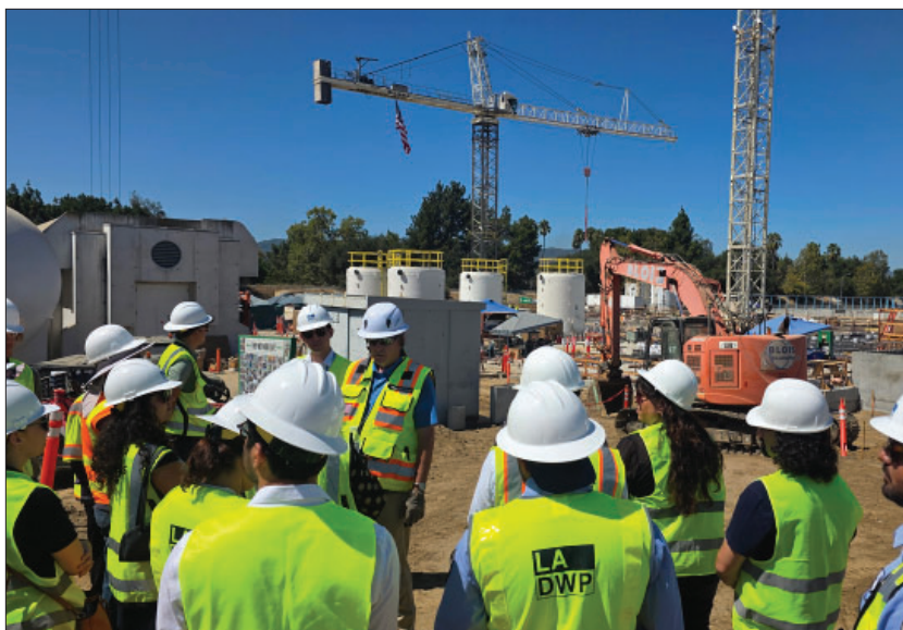
Construction of the LA Groundwater Replenishment Project at the Tillman Plant is set to launch production of 50,000 acre-feet of water annually starting in 2027, more than three times what DWP currently diverts from Mono Basin streams.
